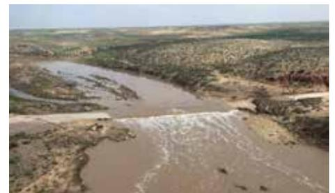
The Pecos River above the Red Bluff Reservoir. Wet areas show how much higher the water had been in the hours prior. It is still flowing a lot of water and has washed out this oil field road. The black poly line you see on the left across the road and on the right in the river bed is an oil field line that used to stretch across the river and as you can see it was separated from the force of the water. Road damage is visible at the current water's edge on both the left and right sides.
