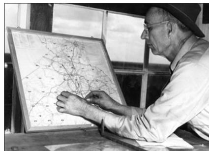
Lookout men used firefinder equipment to most accurately pinpoint locations of possible wildfires. The lookouts would plot the direction of the smoke on a map and contact two other adjacent towers to receive the smoke direction from their locations. With these three plots, they triangulated the approximate smoke location and dispatched fire suppression crews.
