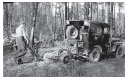
Back in 1950 new technology and more efficient means were developed to help combat wildfires. TFS crew leaders Surcey Peoples and Bob Williams demonstrate how to use a Jeep equipped with a fire plow. They also used a drip torch to set a backfire and remove any flammable fuel near the plowed fire lane.
