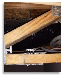
The cause for this metal plate connection to pull out of the bottom chord is unknown, but it is a concern that should be addressed.
