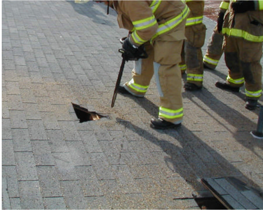
Example of an inspection cut
