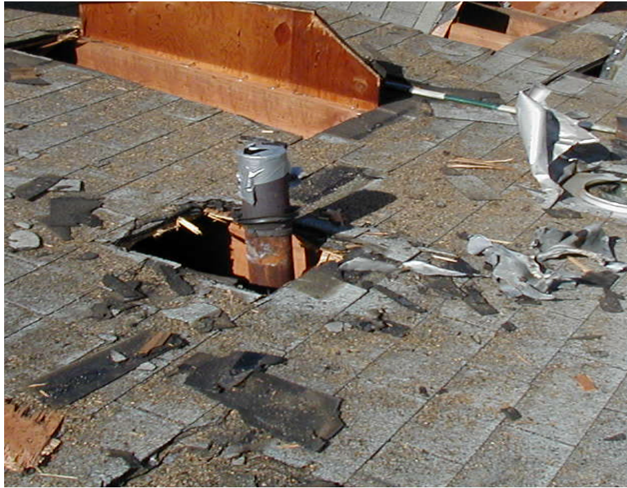
Opening up around the soil pipe.
