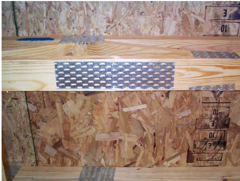
Gusset plates on parallel chord trusses.
