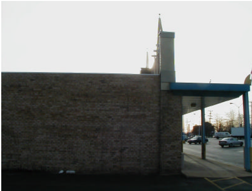
Parapet protruding above the front wall of a shopping center.
