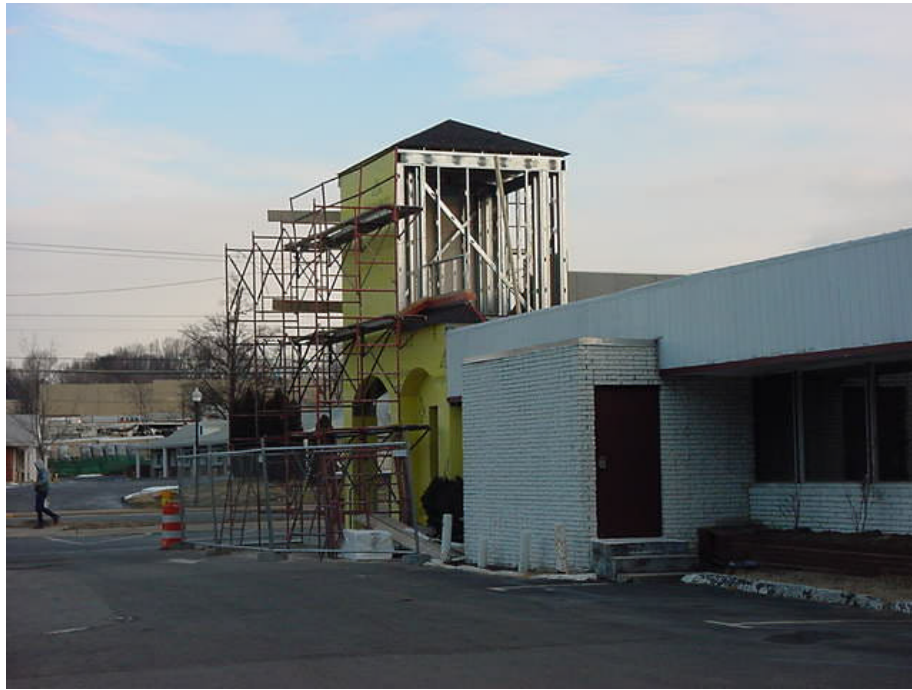
Façade being added to existing structure.
