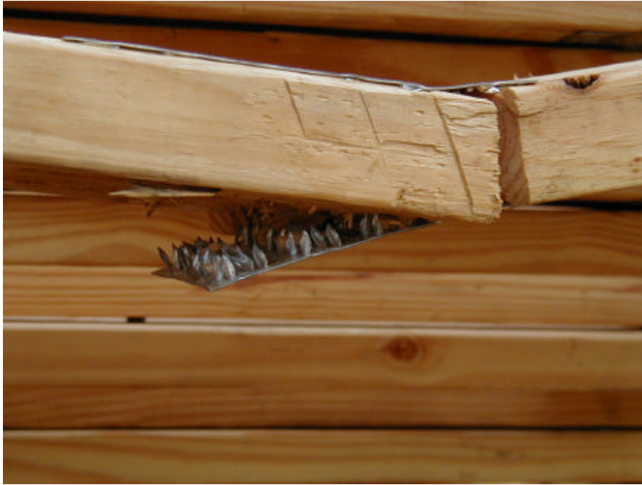
Example of a gusset plate that has pulled away from truss members.
