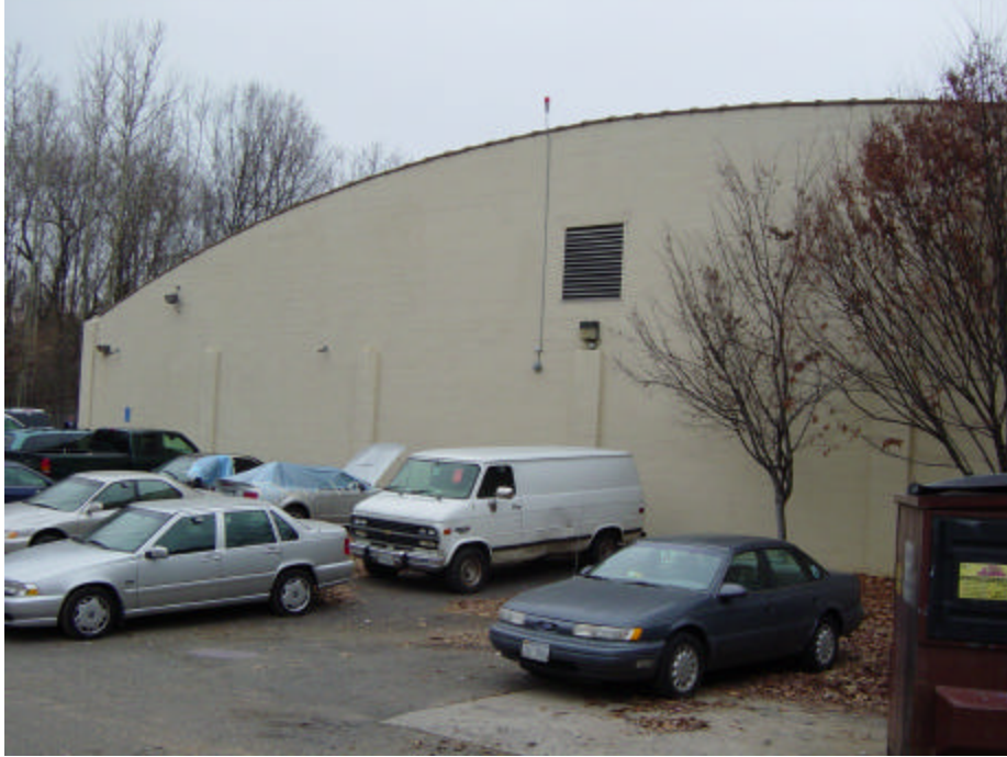
Roof supported by a bowstring truss system.
