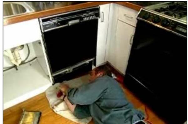
The receptacle for a cord-and-plug-connected dishwasher cannot be located behind the dishwasher.
