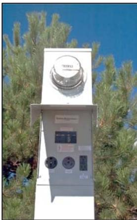
The new definition means that listed electrical equipment can stand alone or it can be mounted on a structure but the listed piece of electrical equipment itself is not considered a structure.
