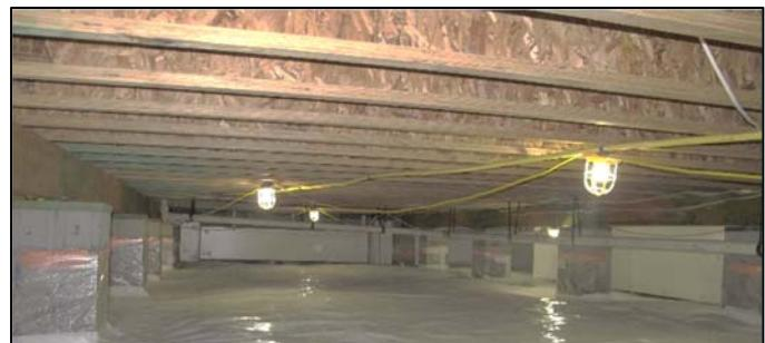
**(E) Crawl Space Lighting Outlets.** GFCI protection shall be provided for lighting outlets not exceeding 120 volts installed in crawl spaces. Fatal incidents have shown amp guards do not provide appropriate shock protection. The GFCI requirement applies to lighting outlets in both dwellings and non-dwellings.
