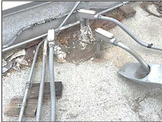
Concerns about separation of conduit when it is used as the equipment grounding conductor and is the sole ground-fault return path brought about a new requirement that outdoor portions of metallic raceway systems that use non-threaded fittings contain a wire-type equipment grounding conductor.
