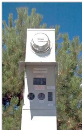
electrode system where all the available electrodes (and if none exist, the made electrodes) are bonded together and to the service or feeder distribution panel. But the existing definition of a structure could include free-standing equipment where the establishment of a grounding electrode system was not intended.
