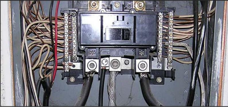
**(1) Location.** Conductors and busbars on a switchboard, switchgear, or panelboard shall be located to be free from physical damage and shall be held firmly in place.
