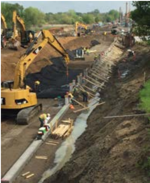
TH 169 Nine Mile Creek Design-Build project
