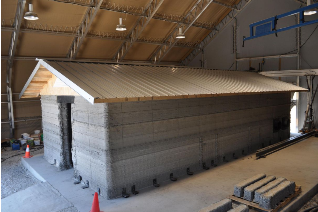
The 512 square feet 3D printed barracks hut (B-Hut), Construction Engineering Research Laboratory (CERL) , ERDC, US Army, Champaign, IL
