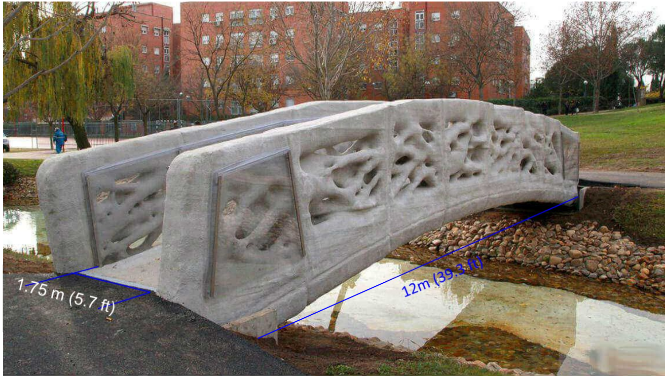
3D Printed Pedestrian Bridge in Madrid (micro reinforced concrete)
