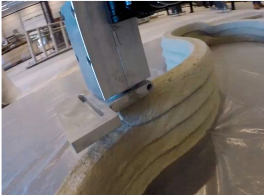
3D concrete printer in operation. No-slump concrete leaves the nozzle as a relatively stiff continuous filament
