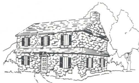
Stone exterior and partial roof between floors
